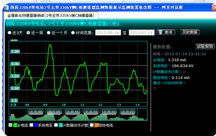
Arrester data monitoring
