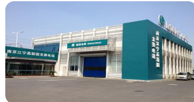
Charging Station of SGCC at Nanning
