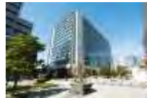
Yokohama Headquarters (Yokohama city, Kanagawa)
